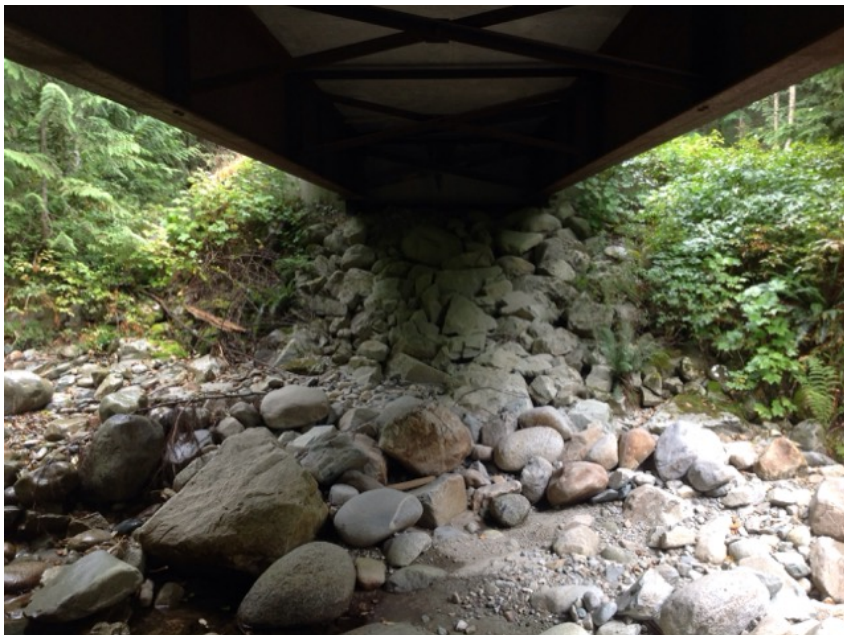
Left Bank Abutment when facing downstream
