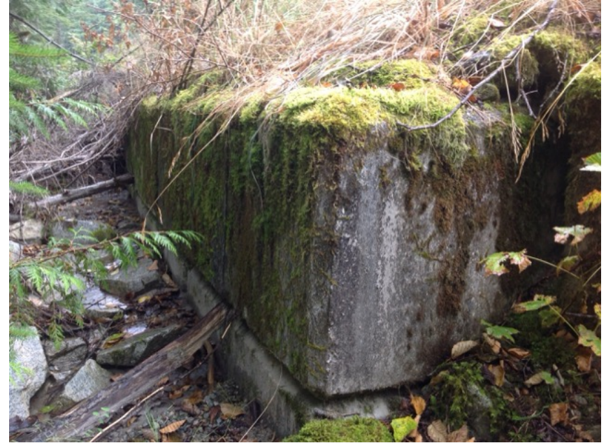
left bank upstream wing wall
