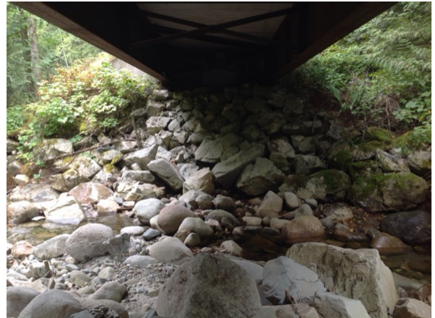
Right Bank Abutment when facing downstream
